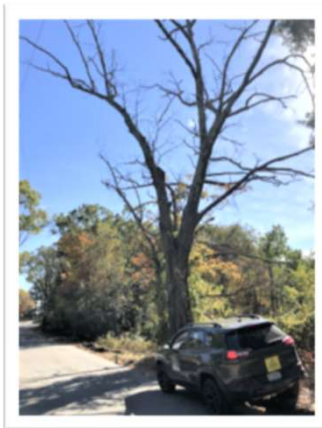
This Image is a Priority 1 dead limb removal due to the proximity over a busy road with the road and wires as a target.
