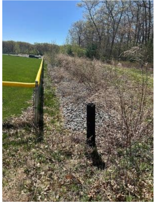
Trench with view port at termination point
