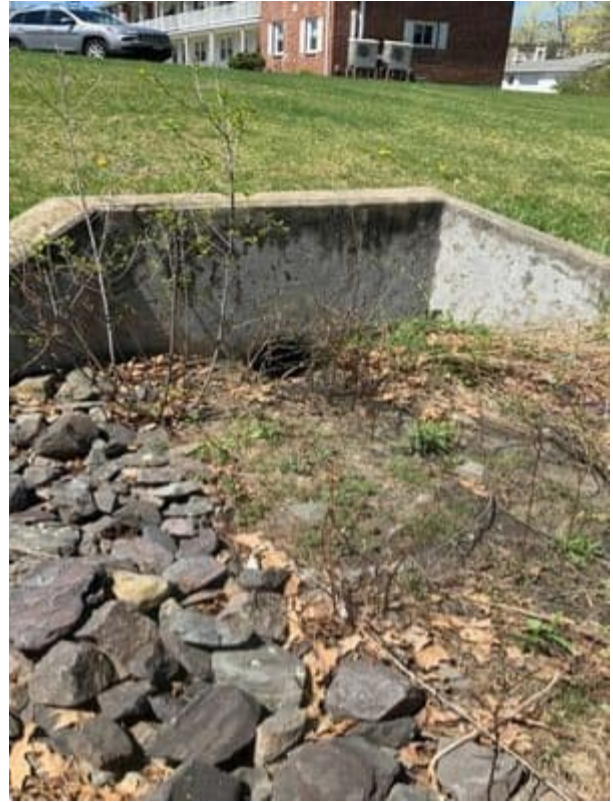
Debris at inlet pipe
