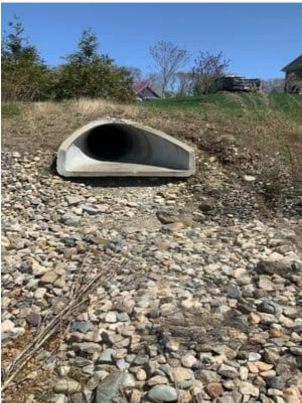
Erosion at 30" outfall into basin
