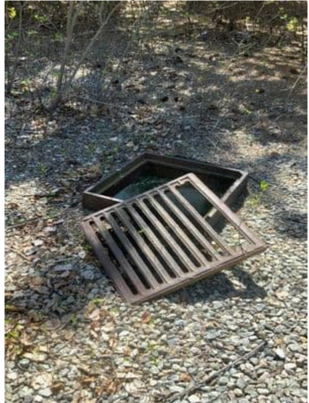
Leaching Catch Basin #4 Cover has been removed and broken. Trash inside catch basin
