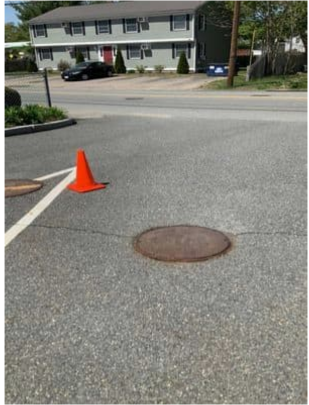
Outside 1st DMH CNO Rusted shut
