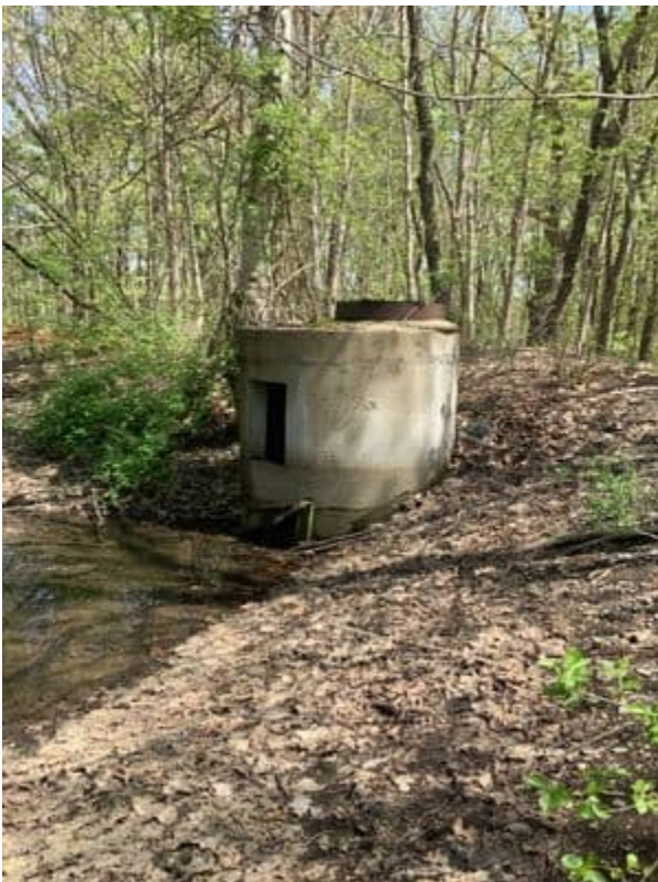
Outlet Control Structure
