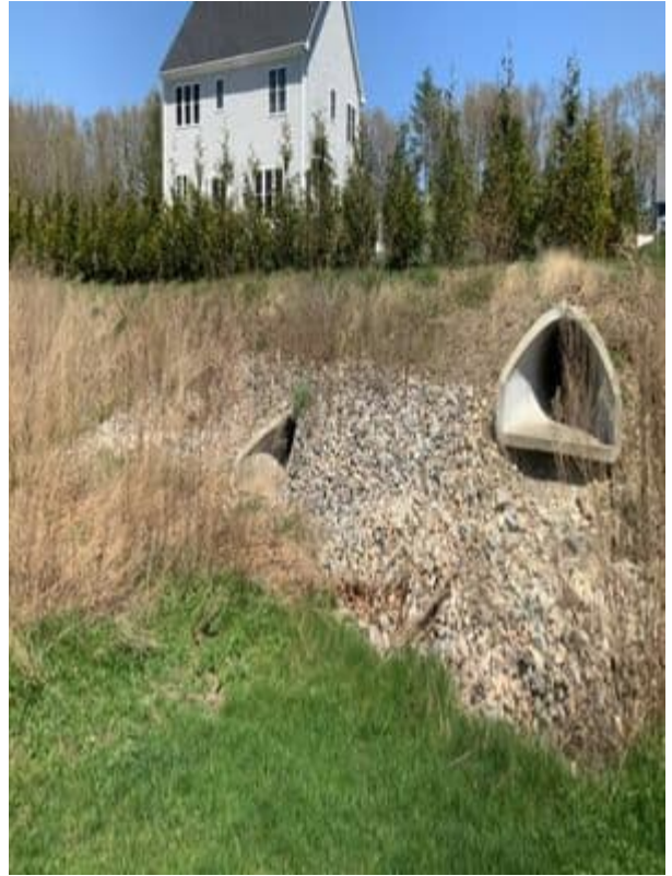
Three basin inlets to detention basin
