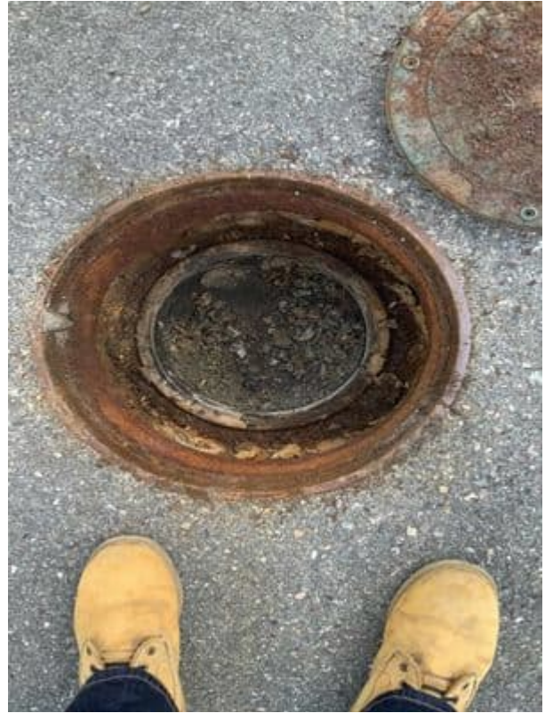
Interior of clean out at handicap parking space
