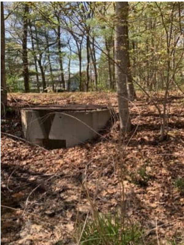
Basin outlet structure
