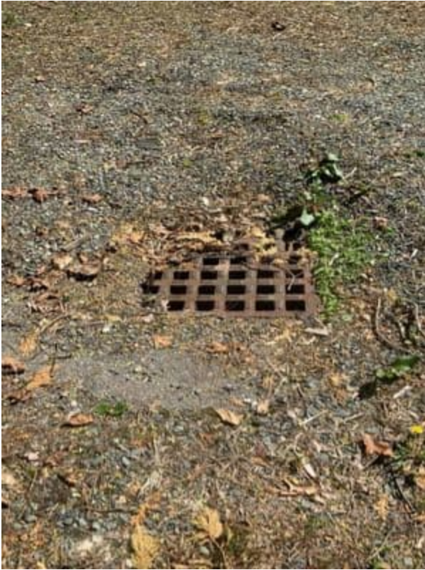
Leaching Catch Basin. Covered in leaves and debris
