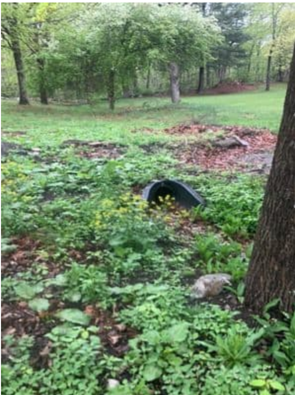
End of basin outlet overland flow to inlet at edge of road
