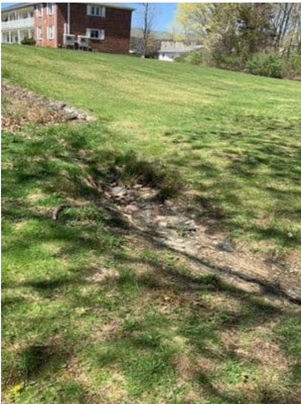
Erosion beyond rip rap channel
