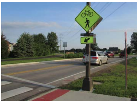
Flashing Beacon crosswalks help alert drivers to pedestrians; these are useful where there are no nearby intersections (FHWA)
