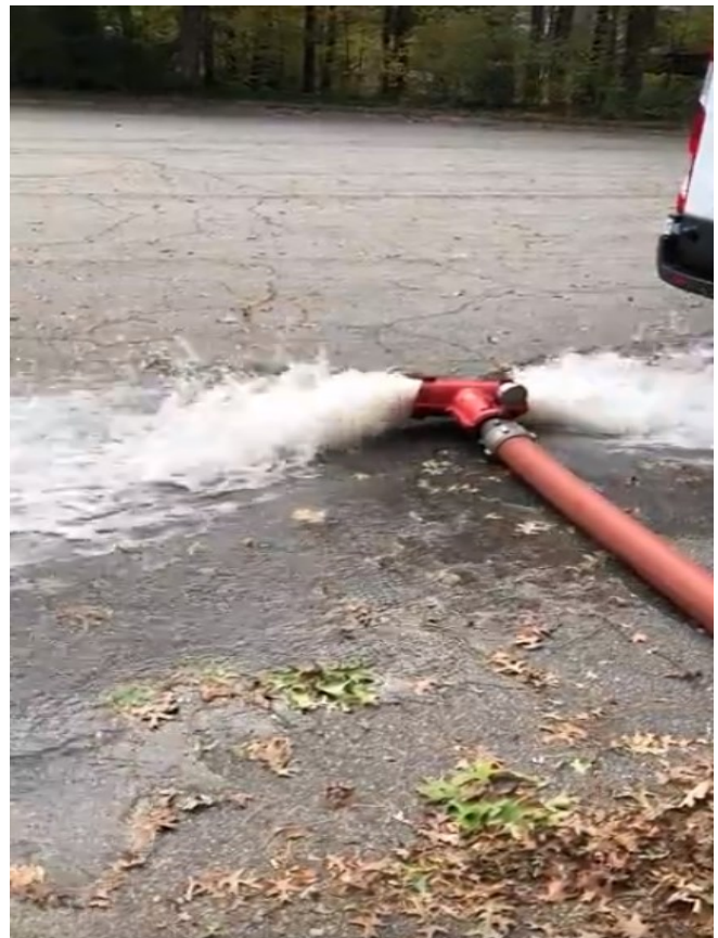
Image of Hydrant Flushing prior to the completion of the Fall unidirectional flushing program
