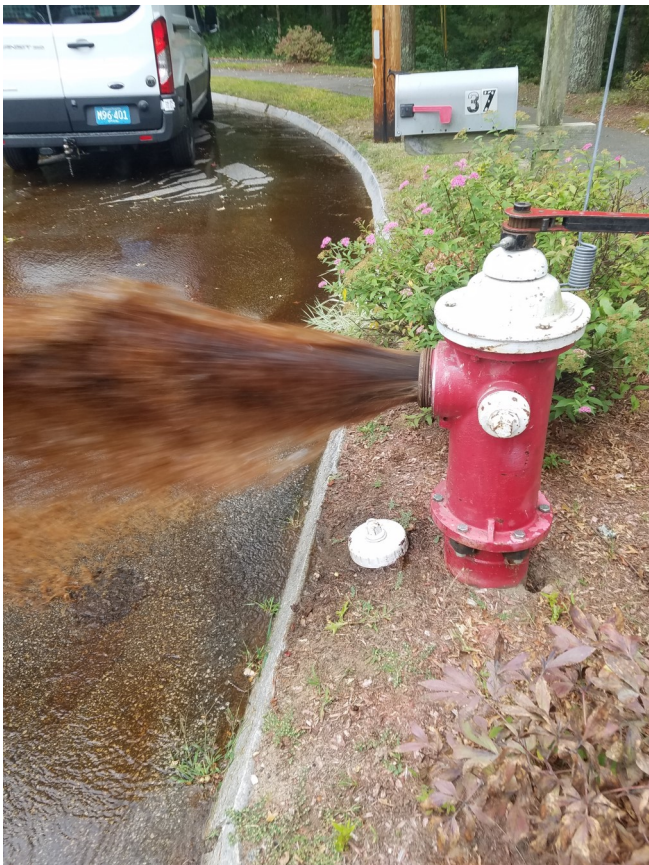
Image of Hydrant Flushing at the Implementation of the unidirectional flushing program
